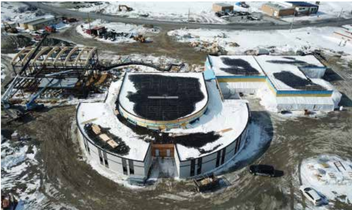
The Youth Healing Centre under construction
